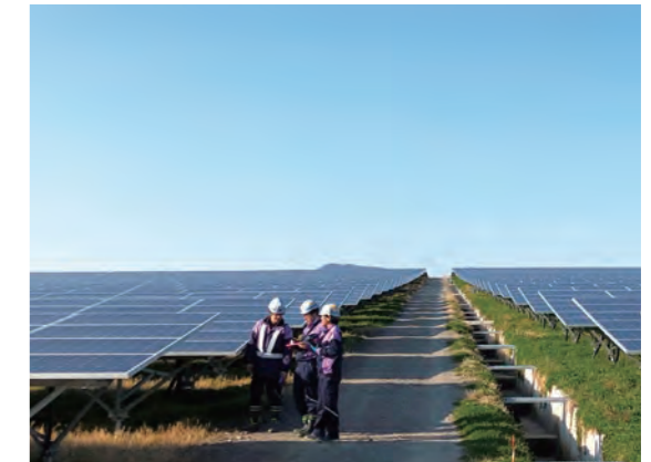
Construction work of a mega-solar system
