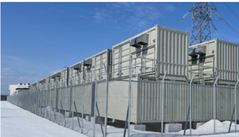
Redox flow battery system for Hokkaido Electric Power Network, Inc.
